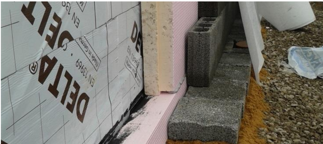
FIGURE 15: XPS PERIMETER INSULATION (CREDIT BY: ©UNIVERSITY OF APPLIED SCIENCES MUNICH)
