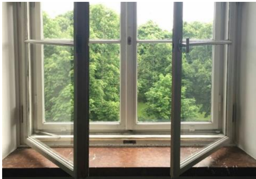
FIGURE 18: SECONDARY GLAZING IN A HISTORICAL BUILDING (CREDIT BY: ©UNIVERSITY OF APPLIED SCIENCES MUNICH)
