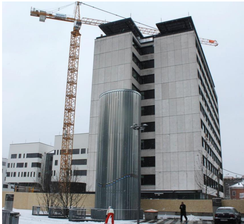
FIGURE 47: LONG-TERM STORAGE INTEGRATED IN THE SHAPE OF THE BUILDING (SOURCE: S. BECKERLE)
