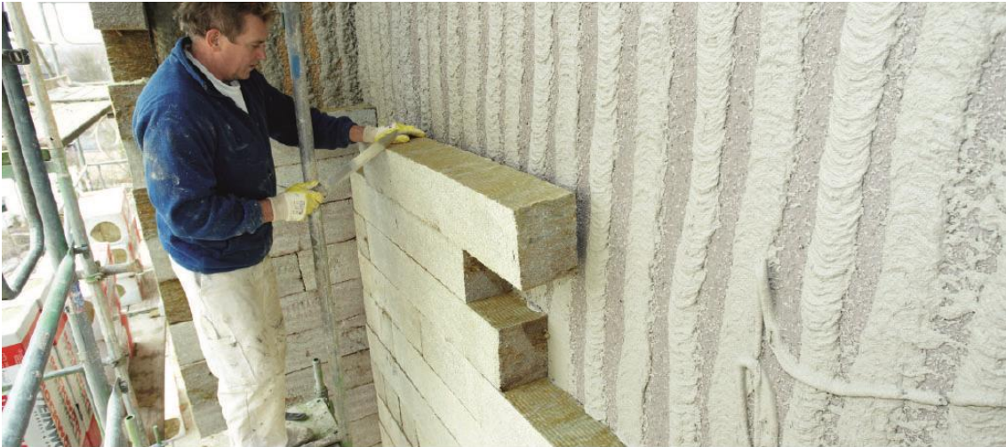
FIGURE 11: INSTALLATION OF THERMAL INSULATION COMPOSITE SYSTEMS (SOURCE: DEUTSCHE ROCKWOOL)
