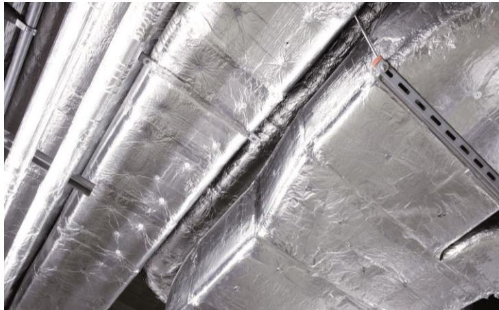
FIGURE 17: INSULATED VENTLAITION DUCTS (CREDIT BY: ©UNIVERSITY OF APPLIED SCIENCES MUNICH)
