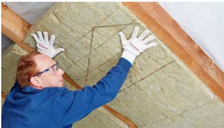
FIGURE 13: BETWEEN RAFTER INSULATION (SOURCE: DEUTSCHE ROCKWOOL)
