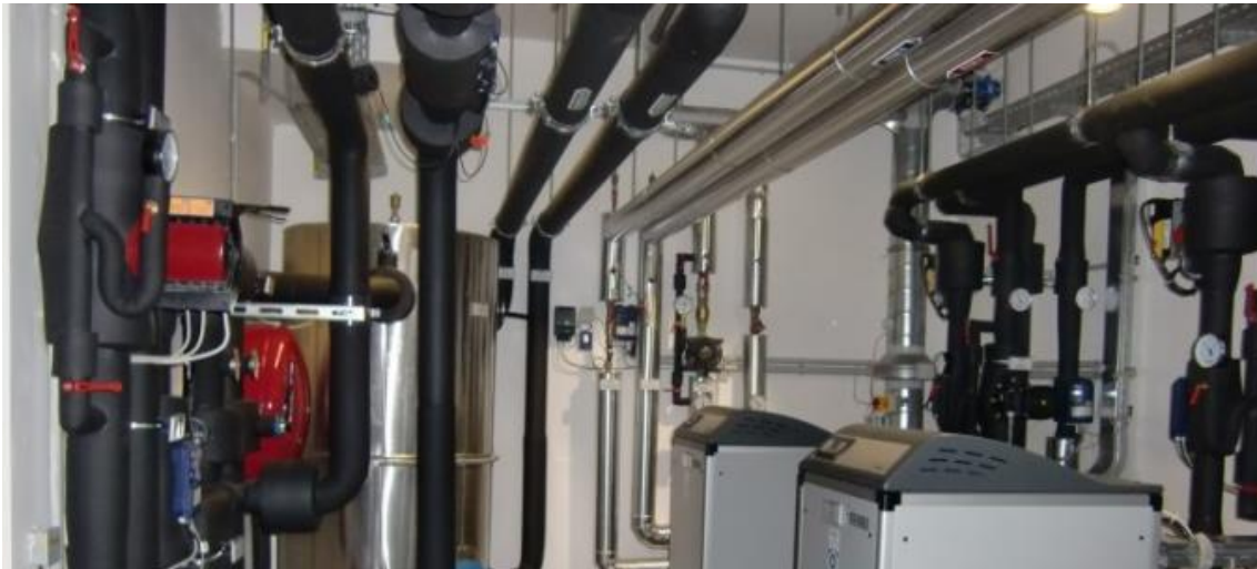
FIGURE 16: INSULATION OF HEATING PIPES (CREDIT BY: ©UNIVERSITY OF APPLIED SCIENCES MUNICH)
