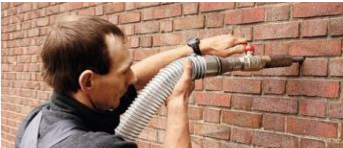
FIGURE 12: CAVITY WALL INSULATION (SOURCE: DEUTSCHE ROCKWOOL)
